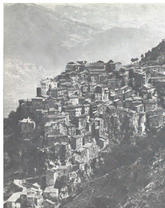
Figura 54. Anticoli Corrado. Imagem retirada de: Rudofsky B. (1964) "Architecture without architects. An introduction to non-pedigreed architecture."
