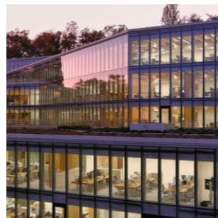
E38| Building H
