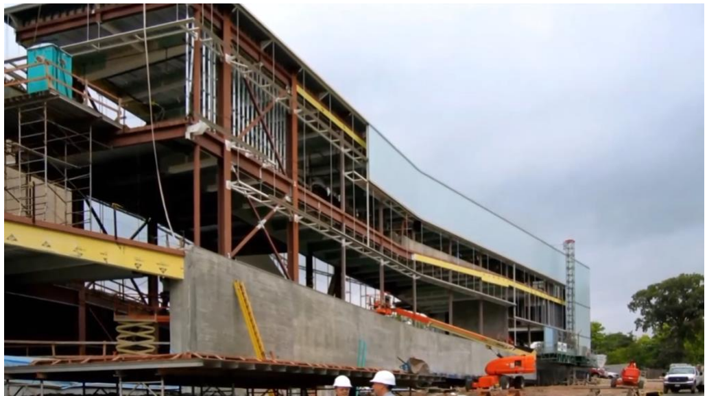
IMG. 151 - Full Segment on the Nelson-Atkins Museum by Steven Holl, Architects (SHELDON, s.d.)
