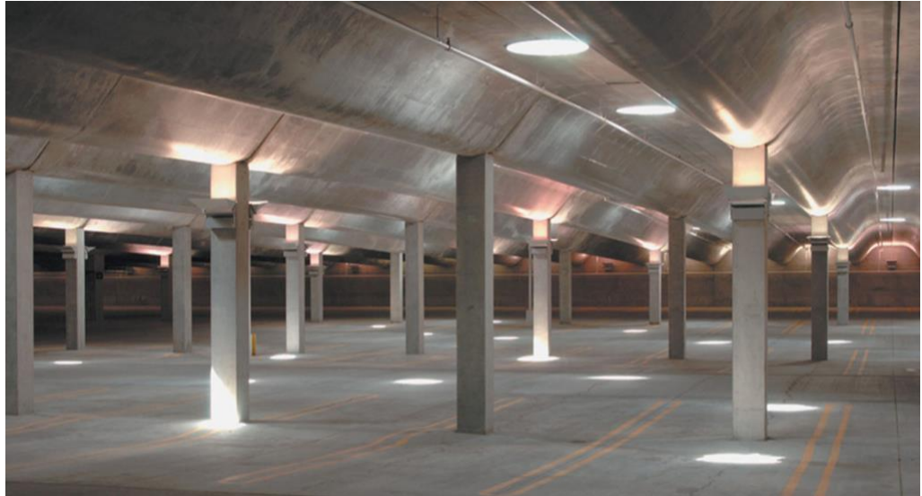
IMG. 160 - Parking garage (RYAN, 2007)
