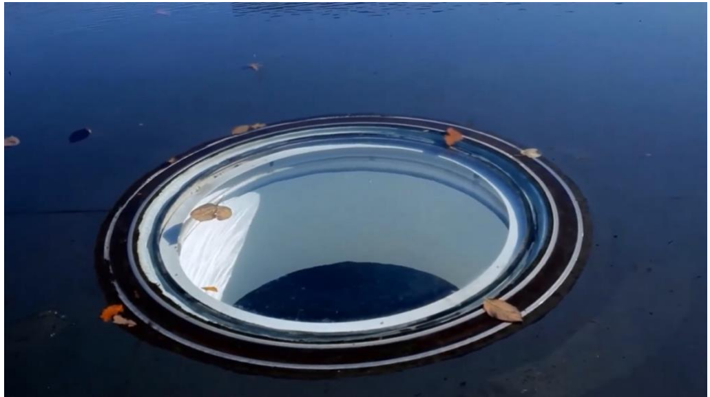
IMG. 157 – Skylights (SHELDON, s.d.)
