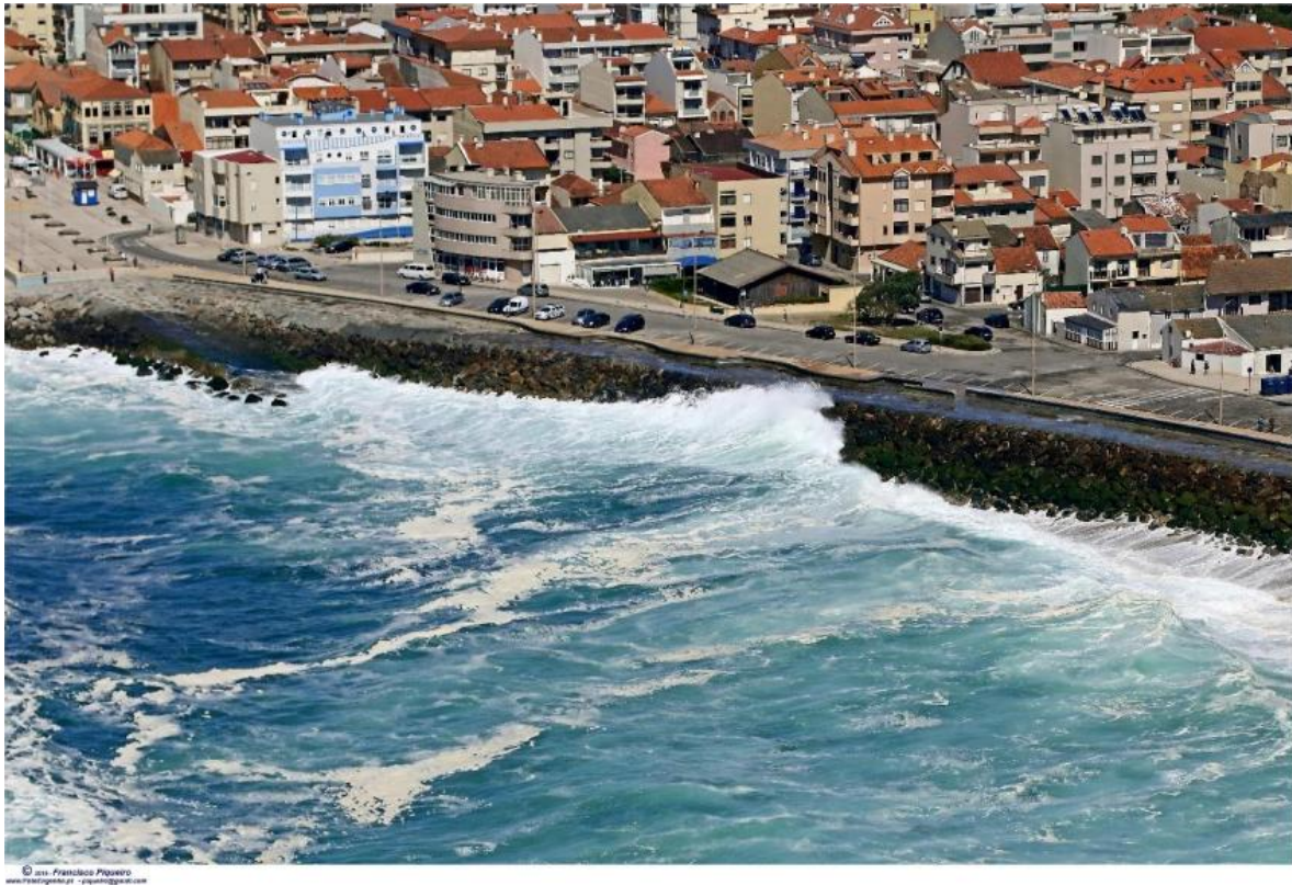
Figure 23 - Zone 2 of Furadouro Beach in Figure 22 – Revetment. (Photo by Piqueiro, 2015)
