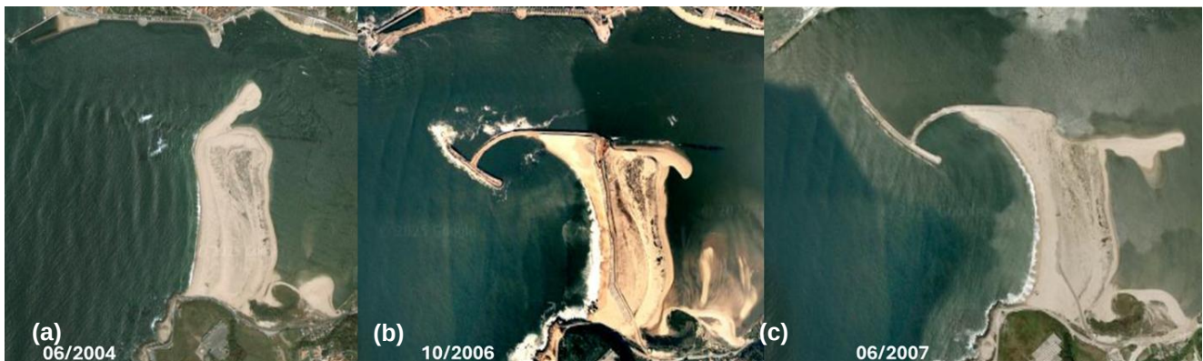
Figure 45 - View of maritime work temporal evolution (2004-2007): (a) Before construction; (b) During construction; (c) After construction (Google Earth).
