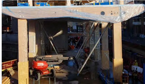
Figure 3. Floor beams during fabrication
