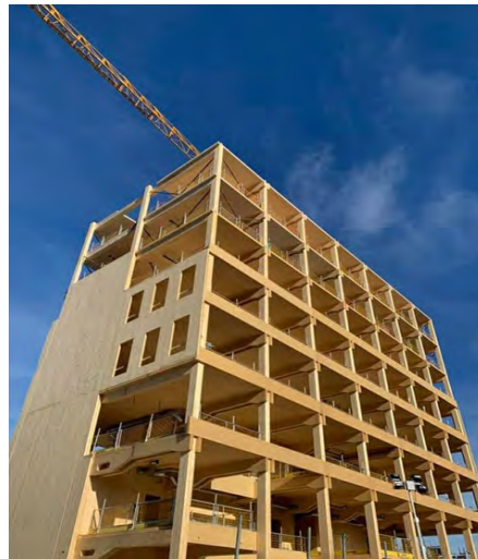
Figure 3. SporX under construction showing the exposed structural frame.
