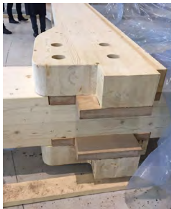
Figure 4. LVL timber transfer structure
