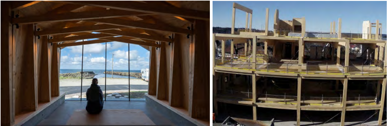
Figure 3. Timber frame buildings – viewing hut and library.
