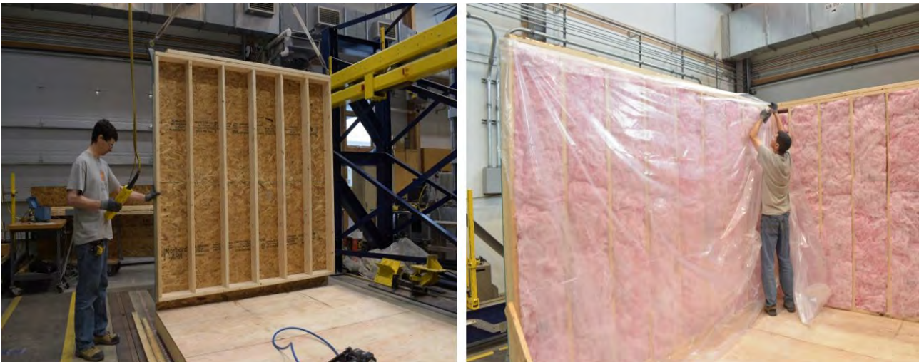
Figure 1. Left, phase 1, prefabrication walls. Right, phase 2, vapor barrier installation
