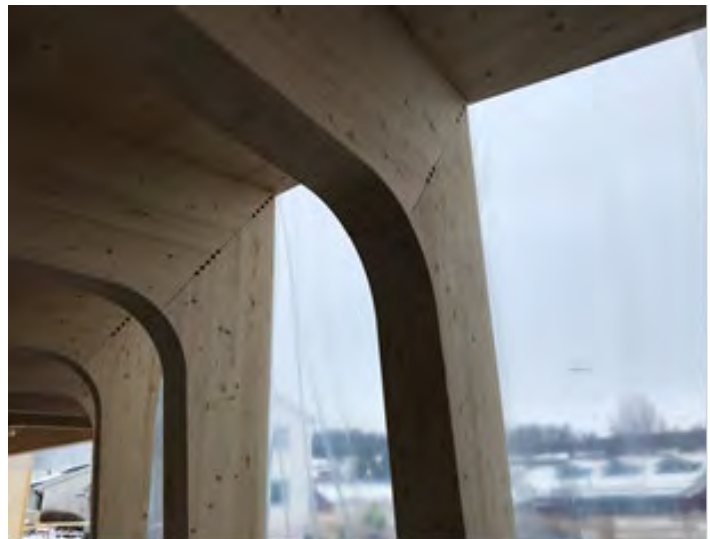
Figure 4. Final aspect of corner joints (©Emma Sukalic)
