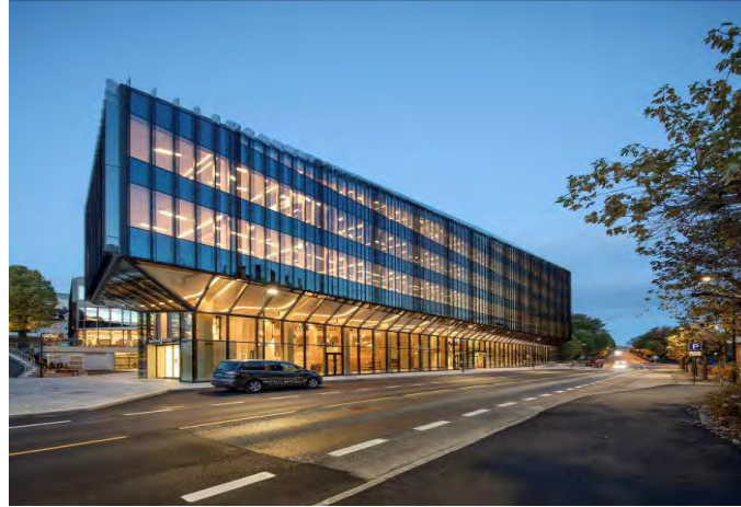
Figure 1. Photo of the finished building (© Sindre Ellingsen)
