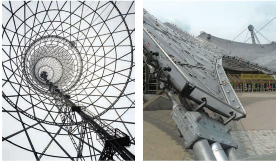
Figure 36, left, Diagrid on Shukhov Tower in Moscow, by Vladimir Shukhov diagrid
