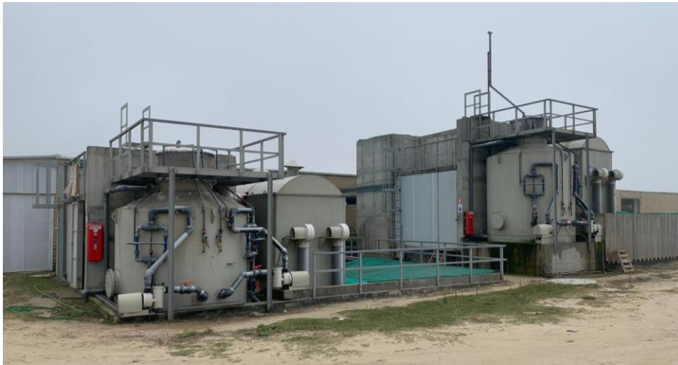
Figure 14 - Pre-Ongrowing's RASs in Safiestela. On the left the RAS from Pre-Ongrowing 1, and on the right the RAS from Pre-Ongrowing 2. Photo taken by Alexandre Veloso.
