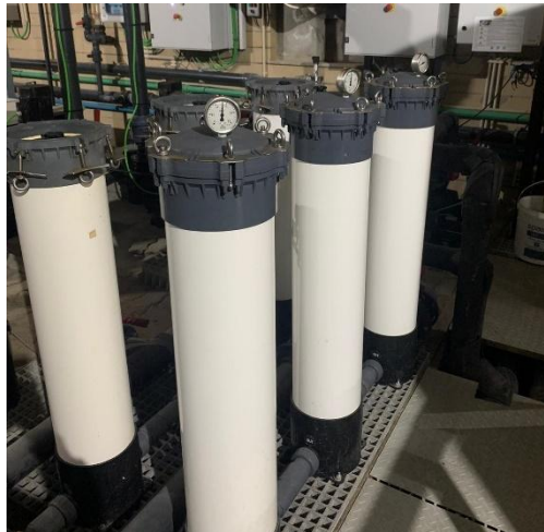
Figure 23 - Cartridge filters utilized in Safiestela to remove impurities from the sea sourced water. Photo taken by Alexandre Veloso.
