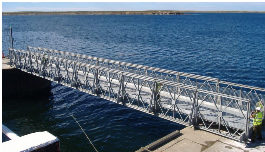
Fig. 2.7 – Ponte pedonal Mabey C200 (adaptada de Mabey Bridge 2023b)
