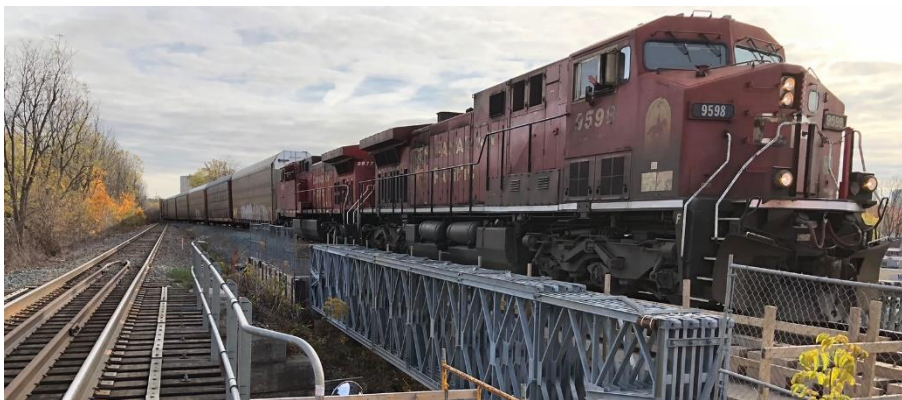
Fig. 2.8 – Ponte ferroviária (Acrow Corporation of America 2023c)
