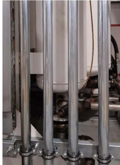
Figure 37- New stainless-steel piping.
