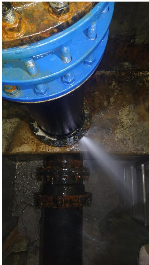
Figure 4 - Joint failure 2
