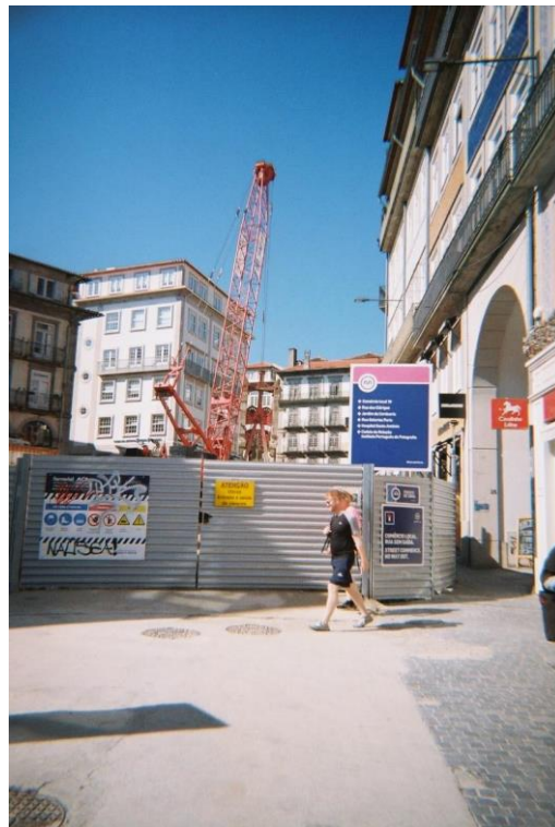
Fig. 10. Photograph by a participant from a deprived non-gentrifying area depicting expansion work on Porto's metro network.
