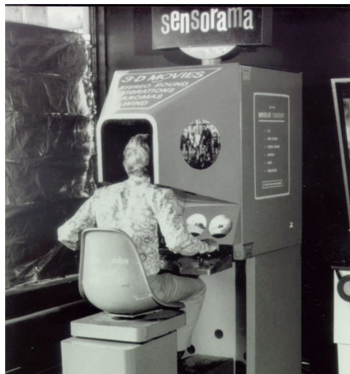
Figure 1.3: First virtual reality device called Sensorama . (Adapted from [22])
