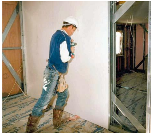
Figure 22 - Attaching plasterboard to the separating wall at X bracing; Source (SCI, n.d.)
