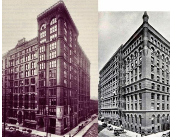
Figure 14 - Rand-McNally Building design by Burnham and Root architects; Source: (Steel Fabrication Service, n.d.).
