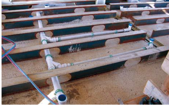
Figure 26 - Inverted Beam; Source (SCI, n.d.)
