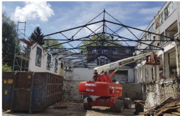
Figure 4 – Deconstruction of building using crane; Source: (Anna Kuehlen et al., n.d.)
