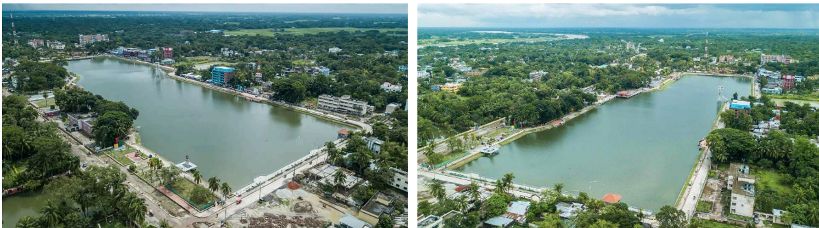
Figure 50 Aerial View of the Shakuni Lake; Source: Vitti Sthapati Brindo Ltd.
