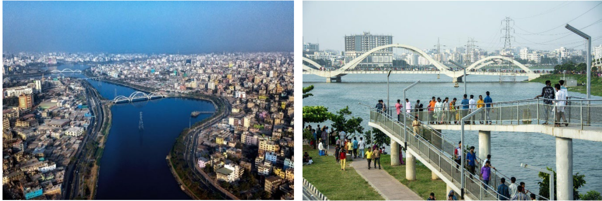
Figure 19 (a) Bird's eye view of the Hatirjheel project; (b) People's activity in the project; Source: Vitti Sthapati Brindo Ltd.
