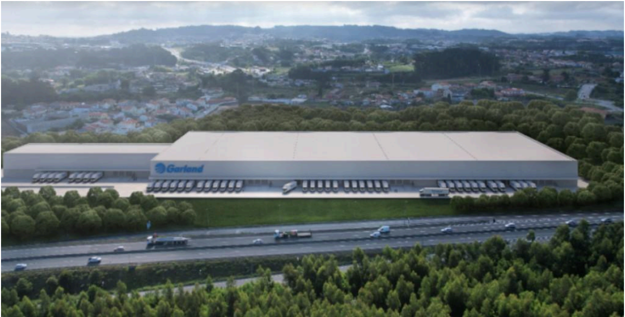
Figure 1 – Facilities of the Logistics Operational Center of Garland Logistics, Lda, located in Vila Nova de Gaia, Valadares
