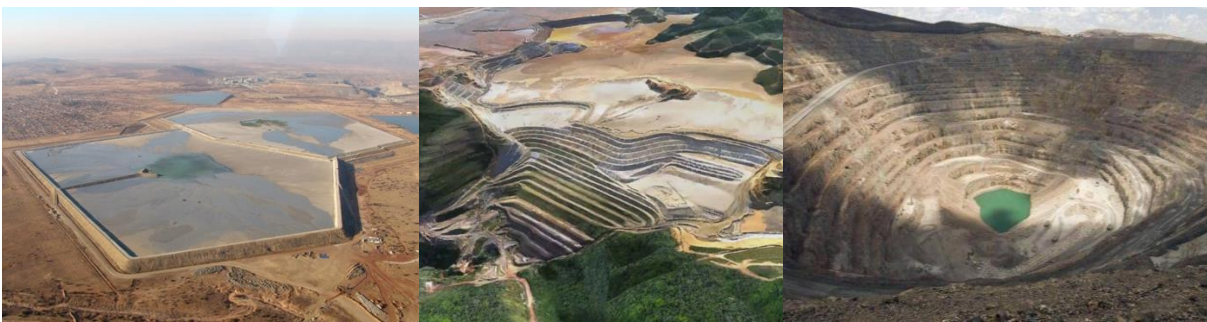
Figure 5 – Conventional tailings storage facilities: a) ring dike - Mogalakwena mine, South Africa; b) valley tailing impoundment - Fundão dam, Brazil; c) in-pit storage – Cadia pit, Australia.
