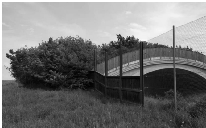
Figure 1.5 - Fences and Screens must be very tightly connected as even small gaps may divert the bats away from the overpass and onto the road. Photo credits: Swild and Nachtkiv
