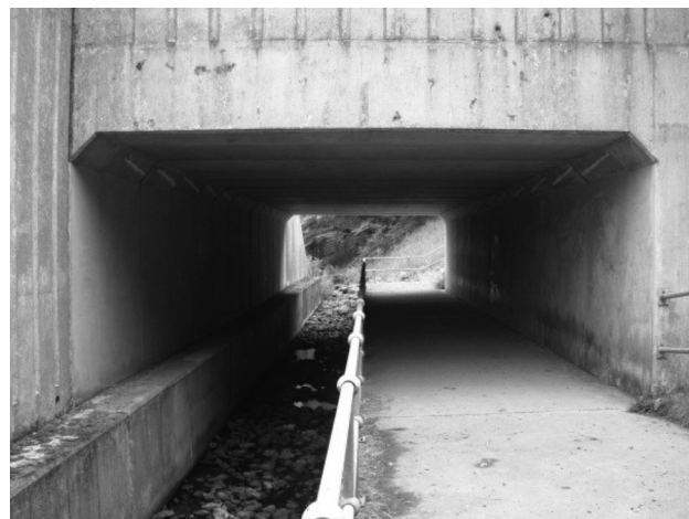
Figure 1.3 - Underpasses on the Agg Cumbria, UK, to guiding bats safely under roads. From Berthinussen and Altringham (2012)
