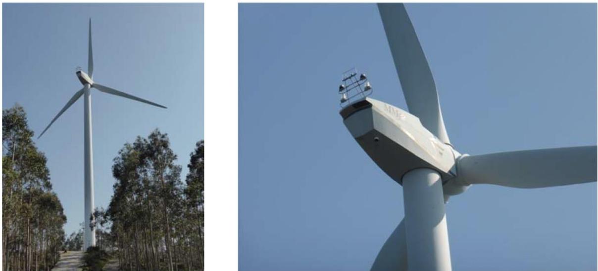
Figure 17 - Wind Turbine under research focus.
