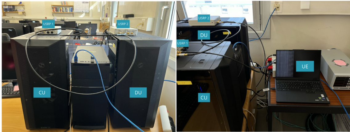
Figure 3.2: Detailed view of the 5G Testbed Radio Access Network (RAN) Components.
