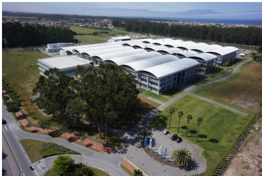
(a) ATEP's facilities.
