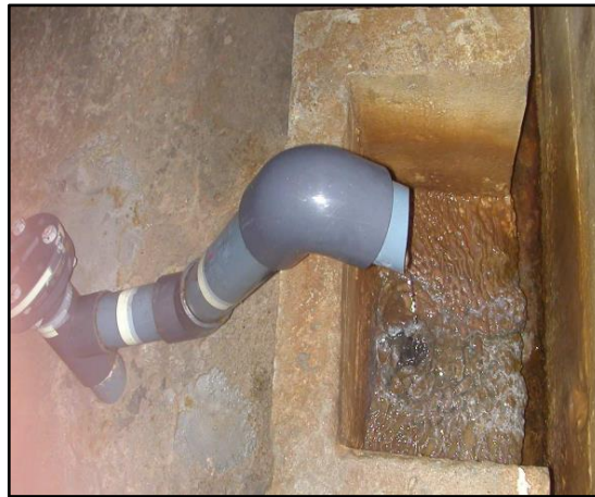
Fig. 10 - Terminal of a drain in a gallery (Moura, 2005).
