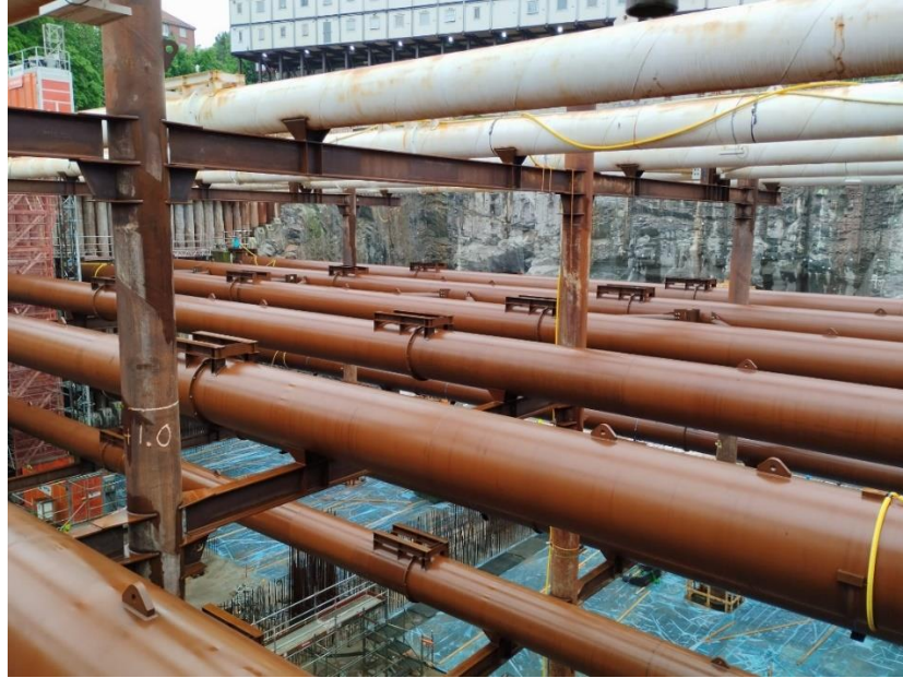
Figure 3.22 – Example of struts used on Korsvägen
