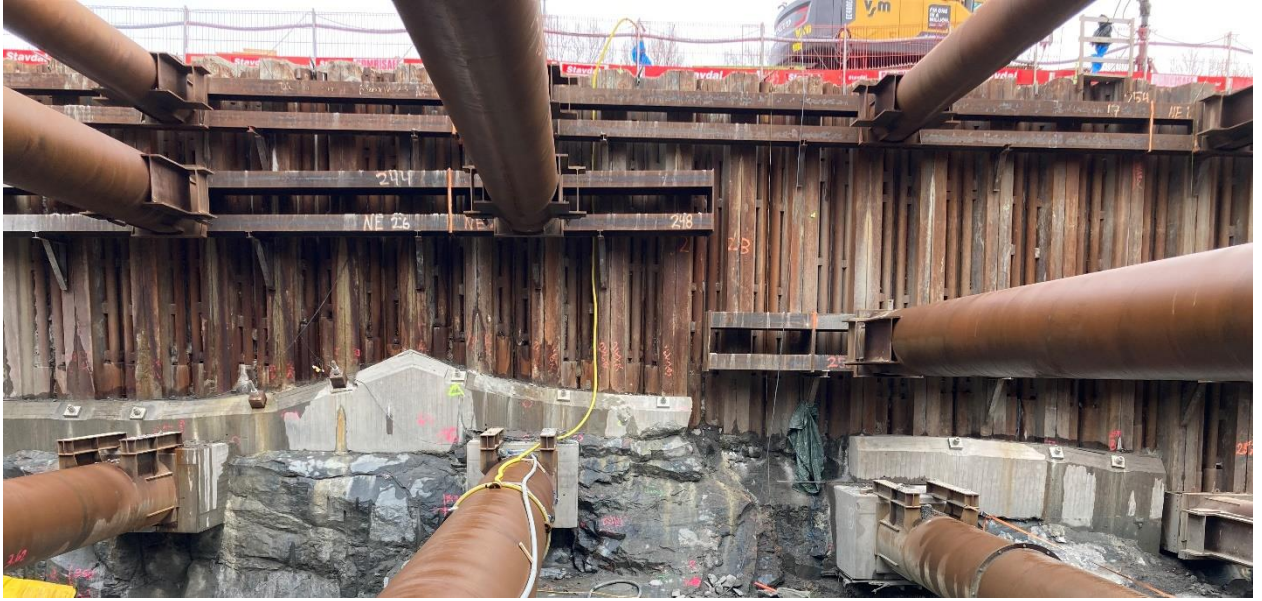
Figure 3.19 – Example of sheet pile wall, Almedal
