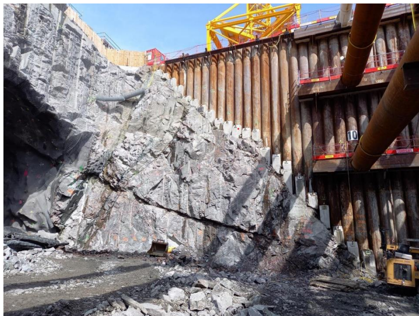
Figure 3.10 – Retaining wall/Rock surface interface, north wall Korsvägen 2 (Kasper T. 2023)
