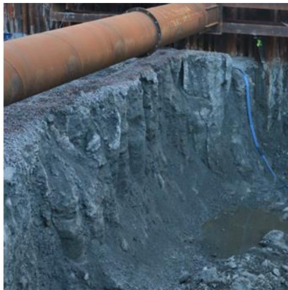
Figure 3.6 – Lime-cement stabilisation
