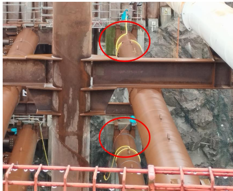
Figure 4.17 – Korsvägen 2 strut row 10 south wall
