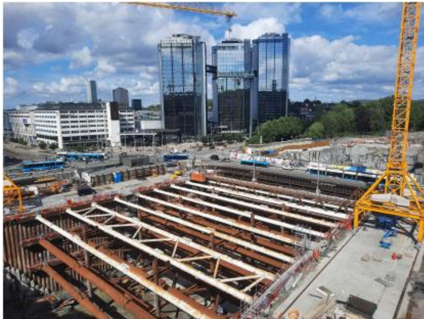
Figure 2.2 – View of the Korsvägen station excavation site (Kasper T., 2023)
