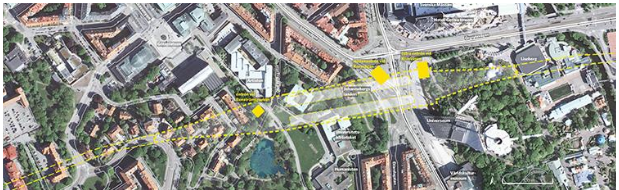
Figure 3.3 – Overview of the Korsvågen construction site (Trafikverket - West Link Project)
