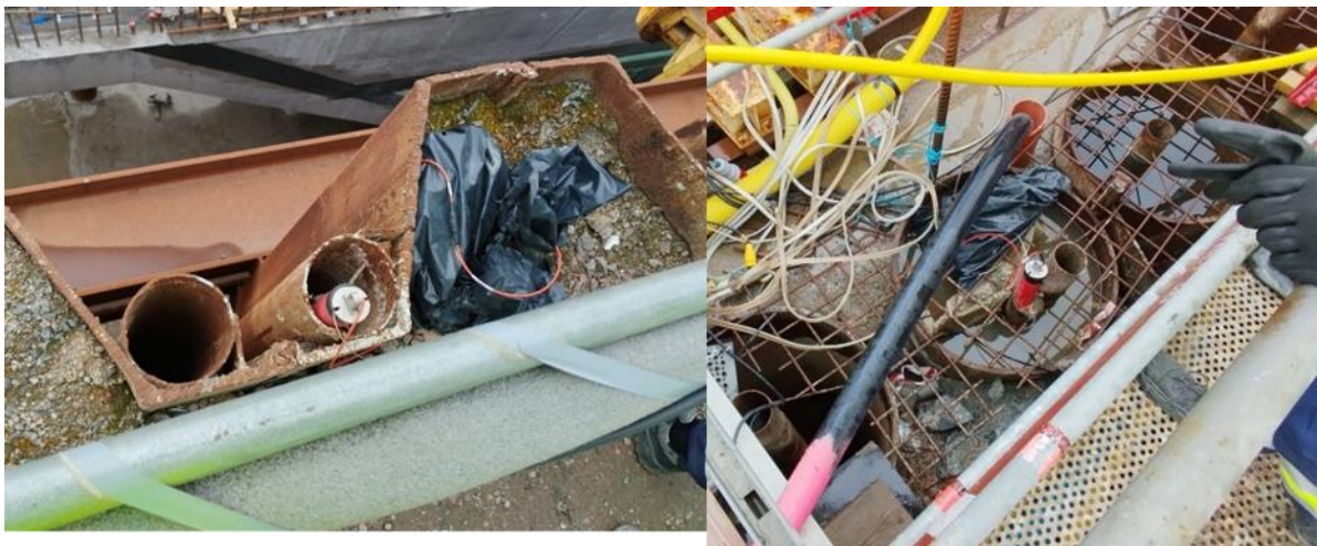
Figure 3.23 – Example of inclinometers, sheet pile (left) and RD pile (right)
