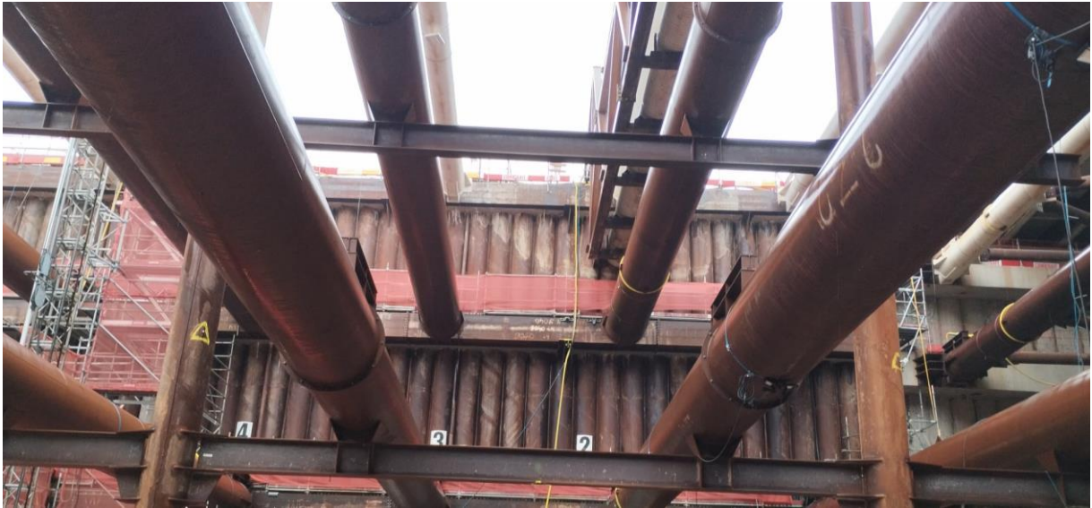
Figure 3.16 – Example of RD piles, Korsvägen 2
