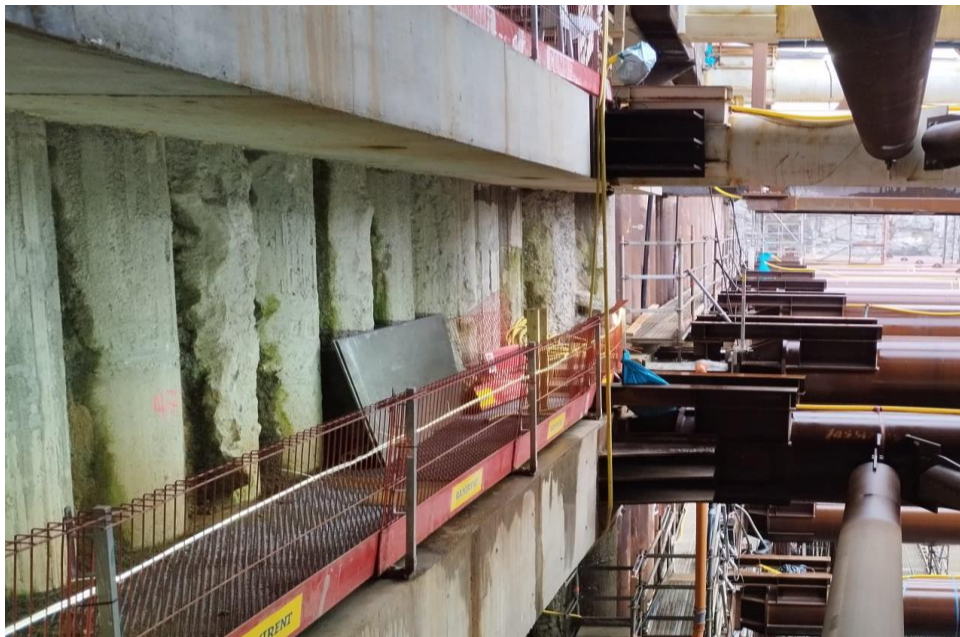
Figure 3.13 – Example of secant piles, Korsvägen 1
