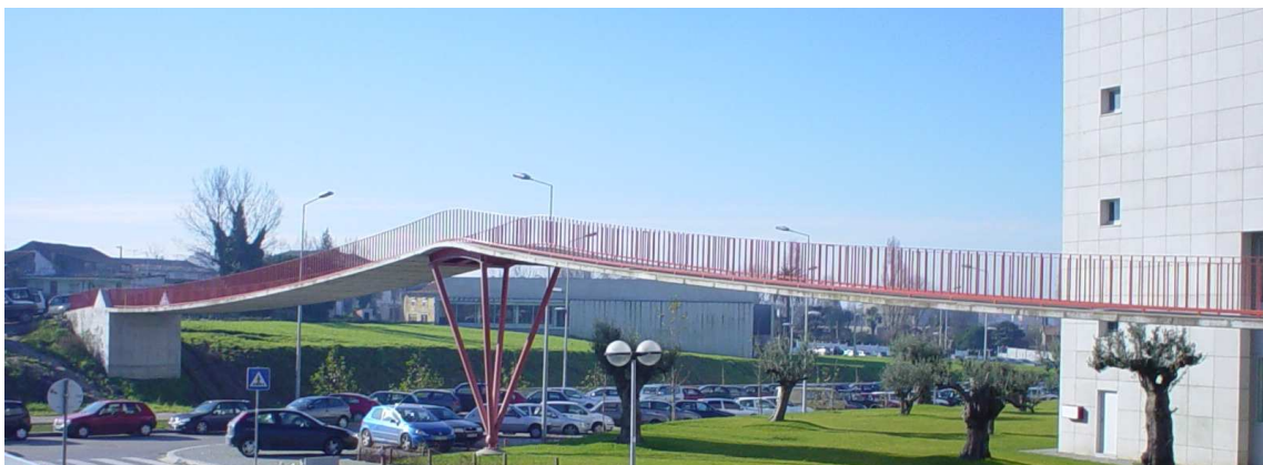
Figure 1. View of the footbridge
