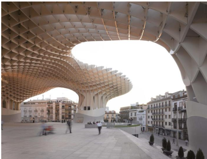
Fig. 84 Cobertura do Metropol Parasol, Jürgen Mayer H. Architects, 2011, Sevilha (Franck, 2011)
