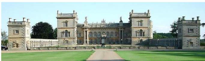
Fig. 17 Fachada a norte do Castelo Grimsthorpe, John Vanbrugh, 1819, Lincolnshire (as-toft.com, 2001)
