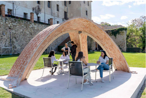
[Figure 22] "innixAR" is an unreinforced masonry structure in Segovia, Spain, built by researches from IE University, Princeton University, and the University of Bergamo which incorporates vernacular and traditional constructions techniques with Augmented Reality, enhancing craftsmanship without the need for physical guides and temporary molds.
