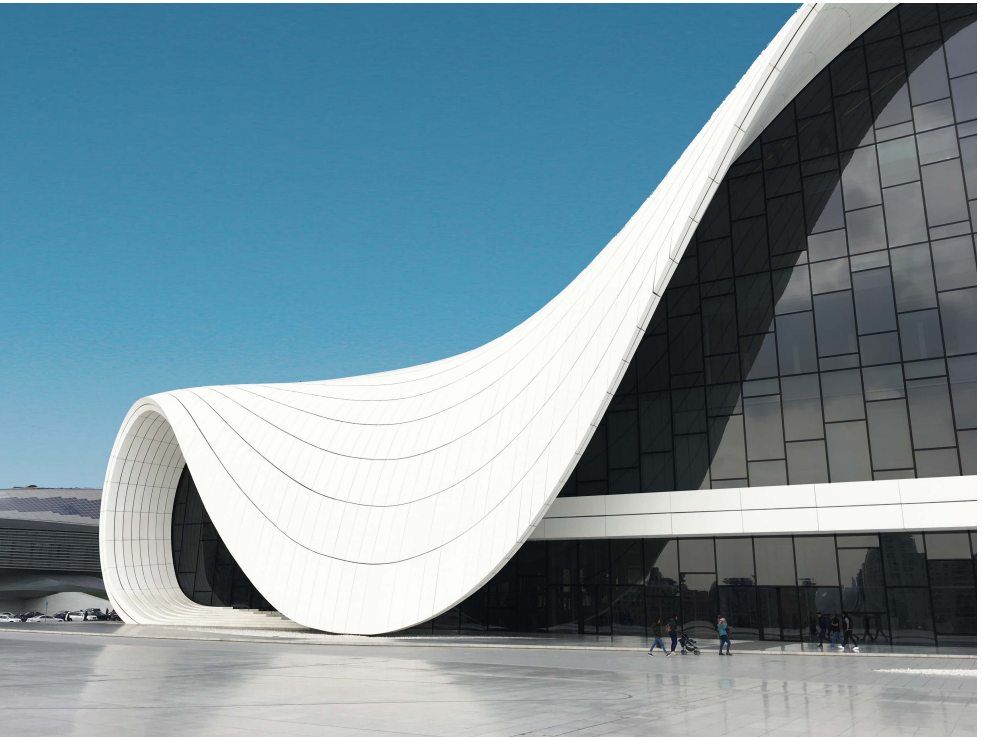
[Figure 104] Removing non-black reflections from the building's glass to increase contrast between the façade's materials.
