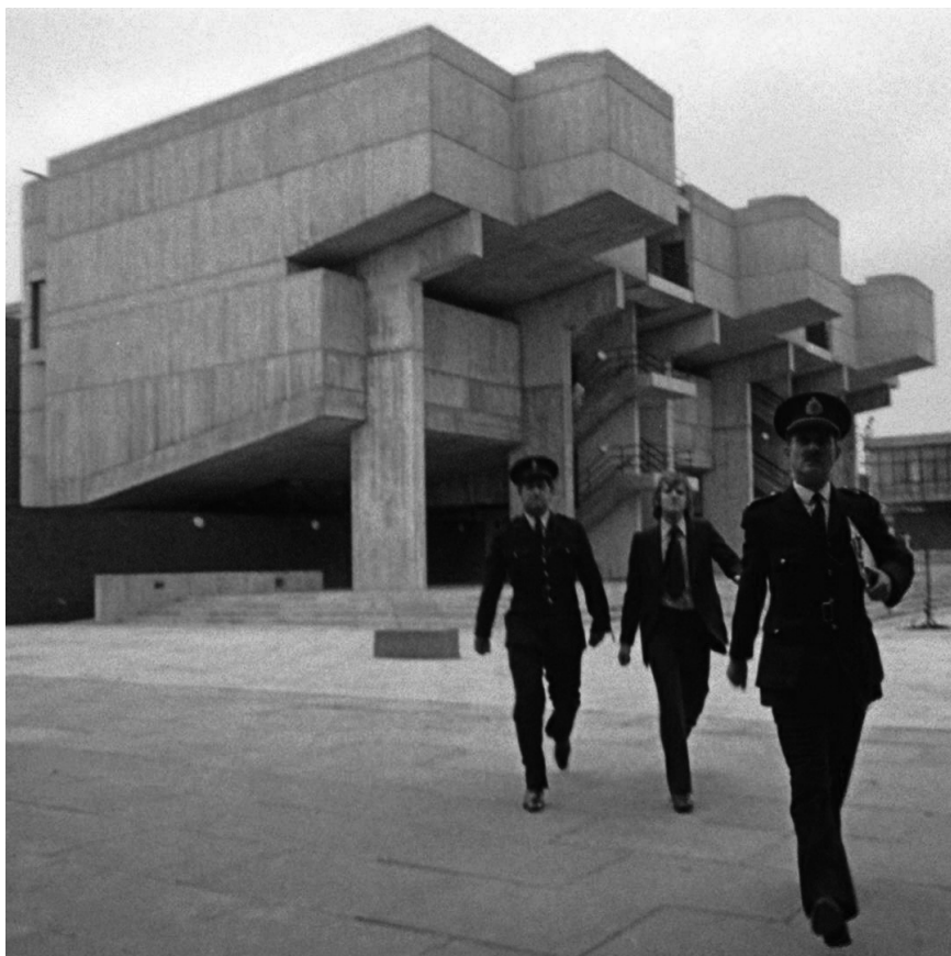
72. Lecture Theatre, Brunel University, Richard Sheppard, Londres, Inglaterra, 1966, em "Clockwork Orange", Stanley Kubrick. 1971
