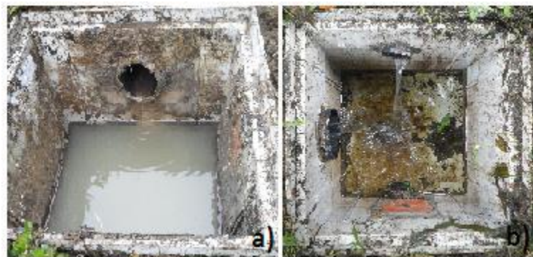
Figure 4 - Sampling boxes at the inlet (a) and outlet (b) of the constructed wetland implemented at Paço de Calheiros.
