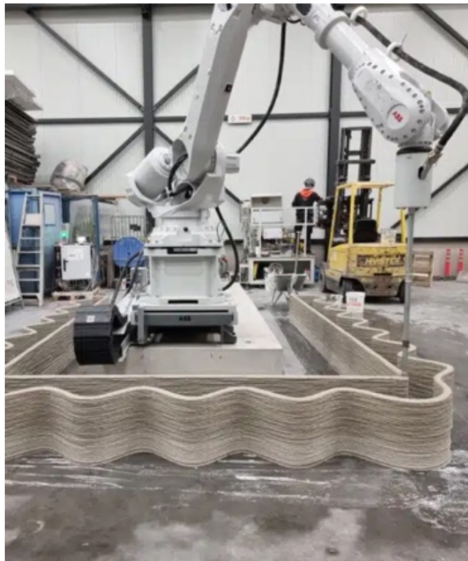
Figure 15. (3D Concrete Printers | CyBe Construction, n.d.)
