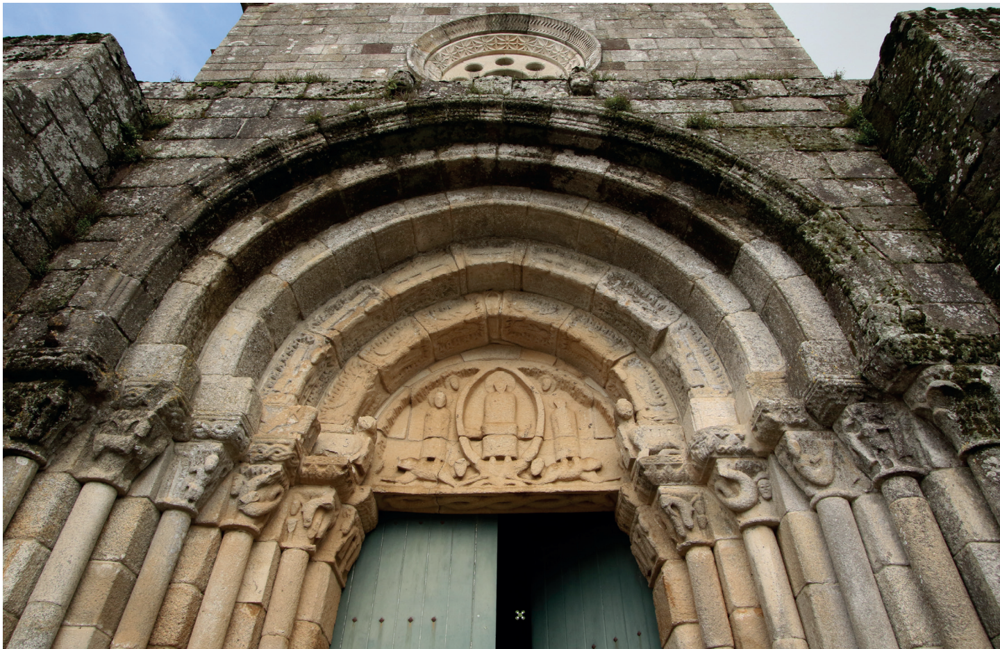
Portal ocidental. Pormenor
