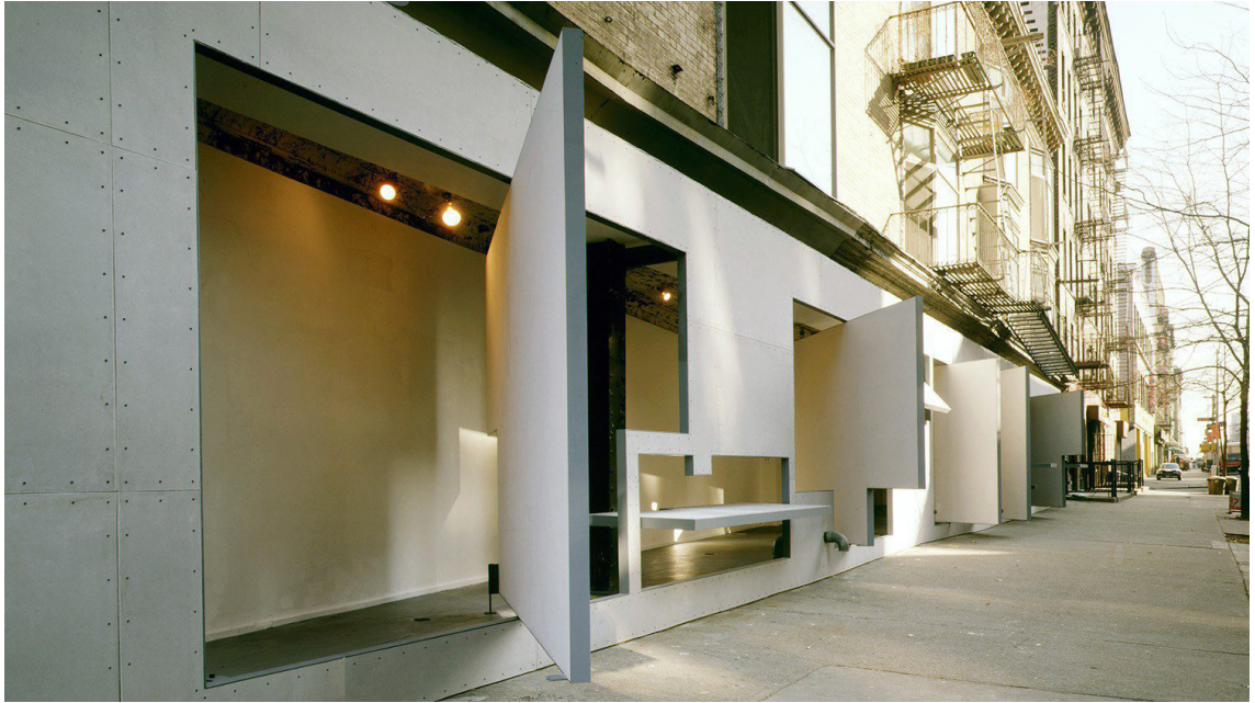
Figura 38 | Storefront for Art and Architecture - Vista Exterior - Steven Holl e Vito Acconci - 1993
