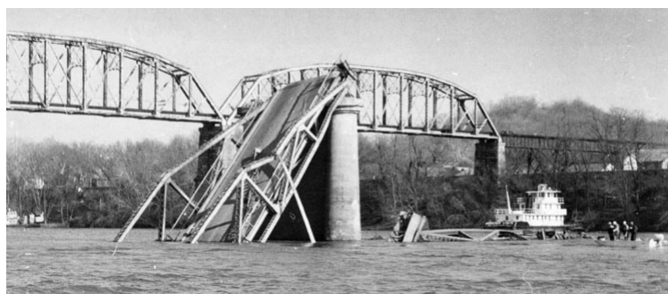
Figure 2.16: Silver bridge after collapse [50]
