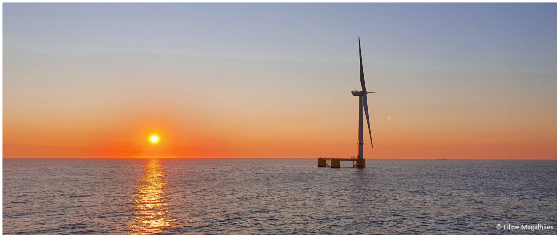
Figure 6.1: Picture of one of the wind turbines from the Wind Float Atlantic wind farm taken during the installation of the monitoring system.
