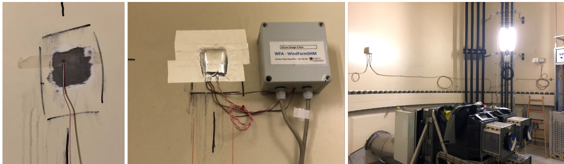
Figure 6.5: Strain gauges' and temperature sensors pictures taken during the installation operation. From left to right: uni-axial strain gauge glued to the prepared tower surface, strain gauge and temperature sensor with protective cover together with connection box and overview of the installation.
