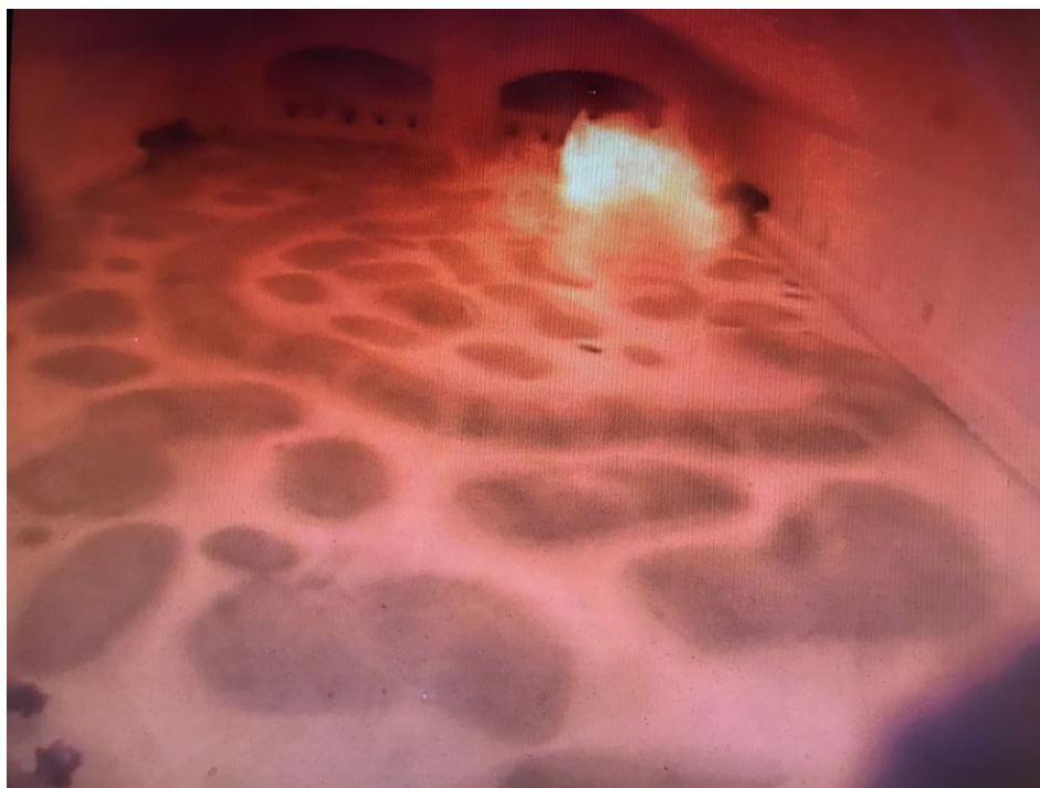
Figure 15 - Flame in the combustion chamber.
