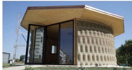
GAIA 3D printed housing project (Shambhala, Italy)
