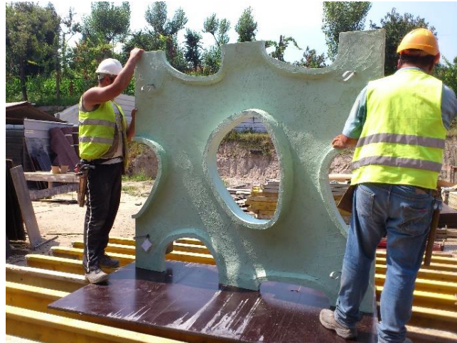
Figura 5 – Painel GRC de geometria complexa
