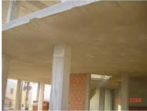
Fig.20 – Laje fungiforme maciça [24]
