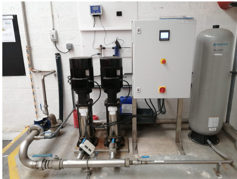
Figure 3.4: EFAFLU AQUA Premium CFD system
