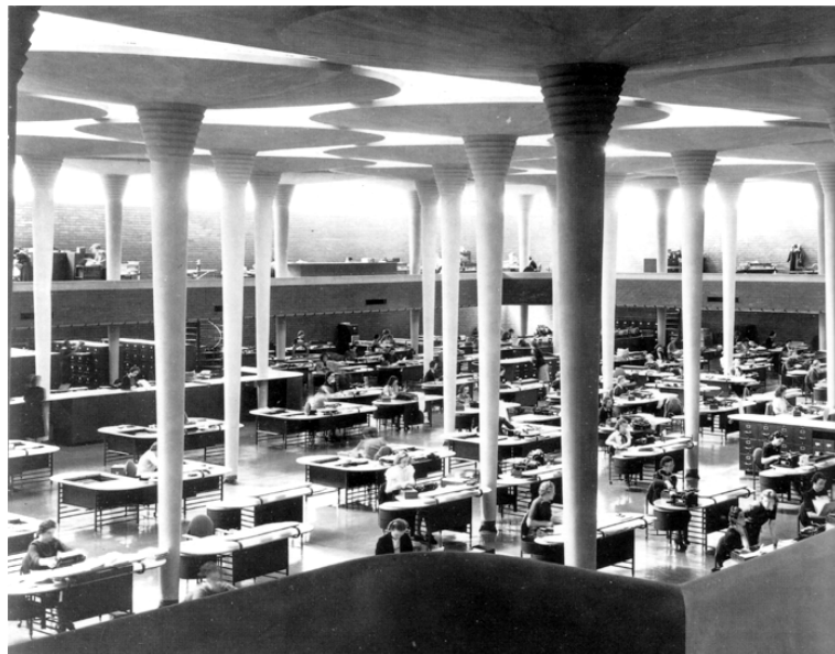
Fig.8 Edificio da Johnson Wax Headquarters, Wisconsin, EU, Frank Lloyd Wright, 1936-39
