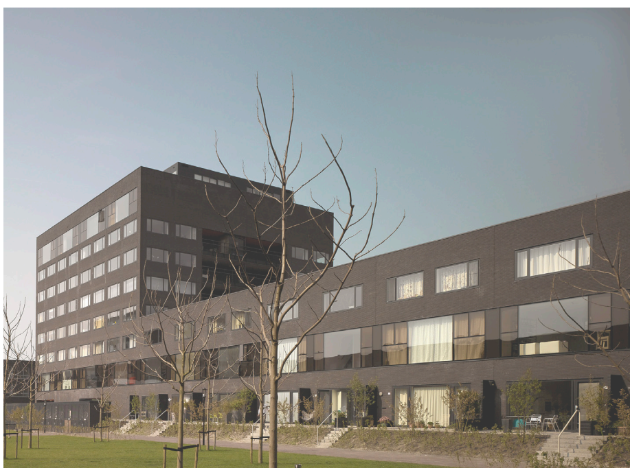
Block 23, Gabinete VMX architects, 1999-2003 fig.109 Fachada posterior
