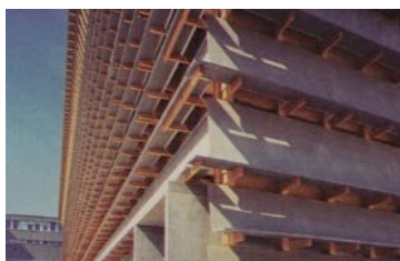
166 | Ricola Storage Building Pormenor
