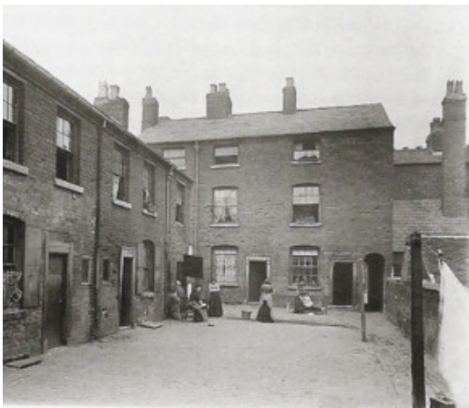
fig.22 [65] "Back to Back Houses" em William Street, Birmingham; 1905.
