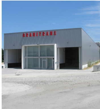
Fig.72: Contentores com front Office.
