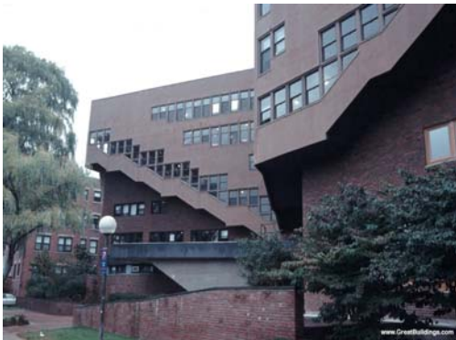
Fig. 105 - Baker House, Massashussets, E.U.A. (Alvar Aalto, 1945 -1947).
