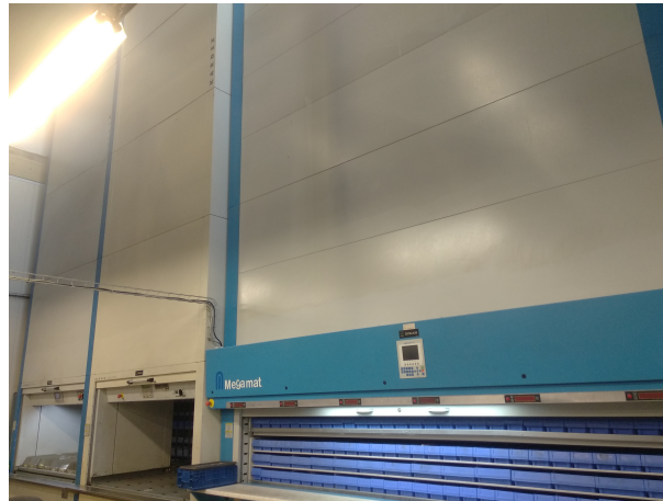
Figure 3.16: 3 of the 4 Vertical Lift Module storage systems
