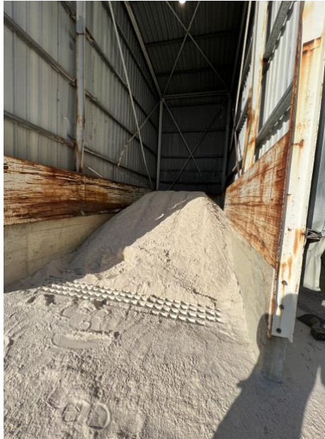
Figure 3.10: Sand unloading site
