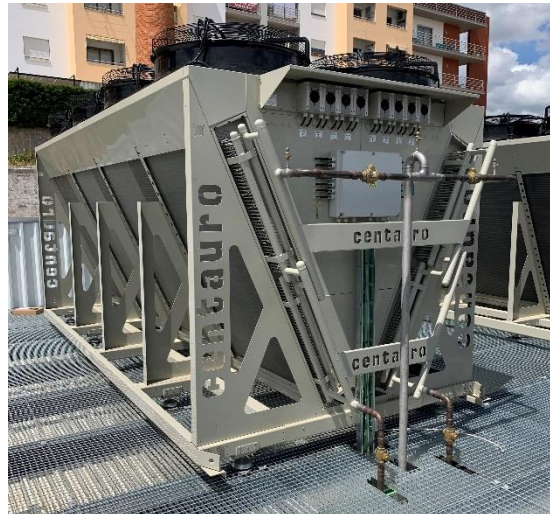
FIGURE 2.18: FORCED CONVECTION AIR COOLED CONDENSER/GAS-COOLER IN A REFRIGERATION INSTALLATION FROM CENTAURO
