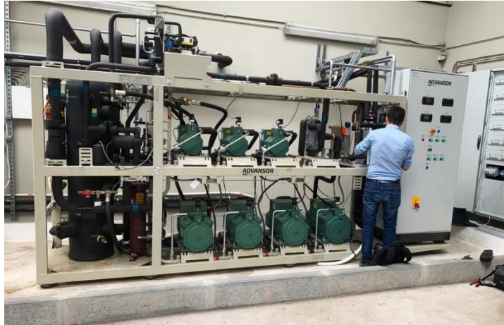
FIGURE 3.1: ADVANSOR CuBIG 3+1x3 CU-1R REFRIGERATION RACK
