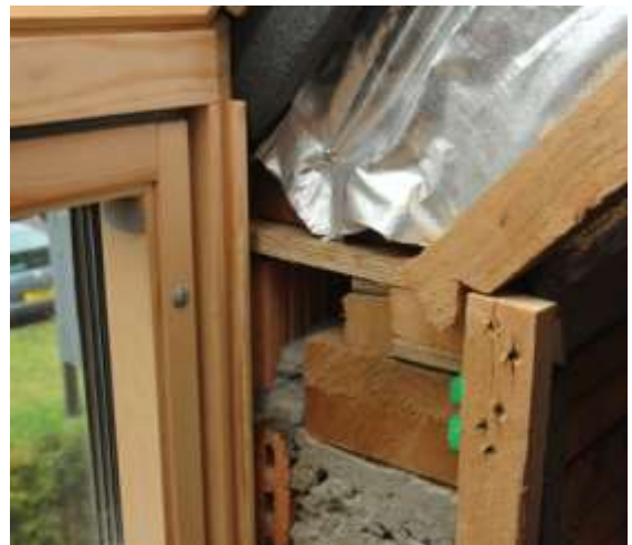
Fig. 3. Real details – typical roof/wall junction.
