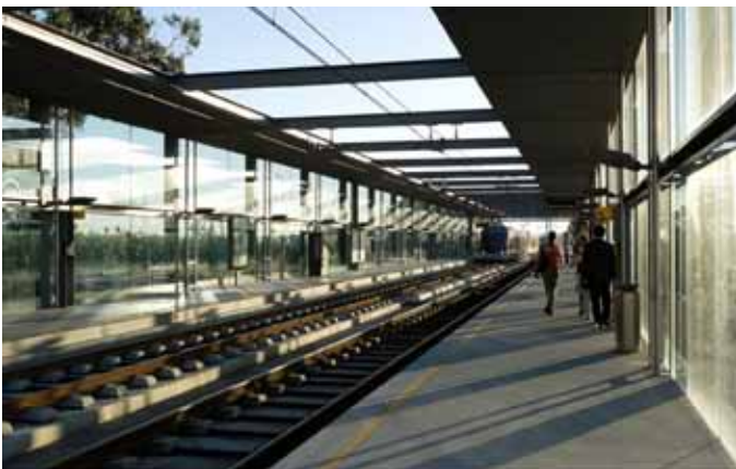
Metro Porto-Parque Maia Station João Álvaro Rocha, Maia, 2001-2007
