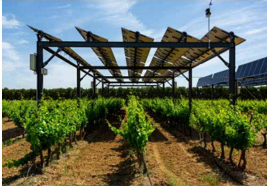
Figure 2.10: OPV wine farm with solar tracking system in France.
