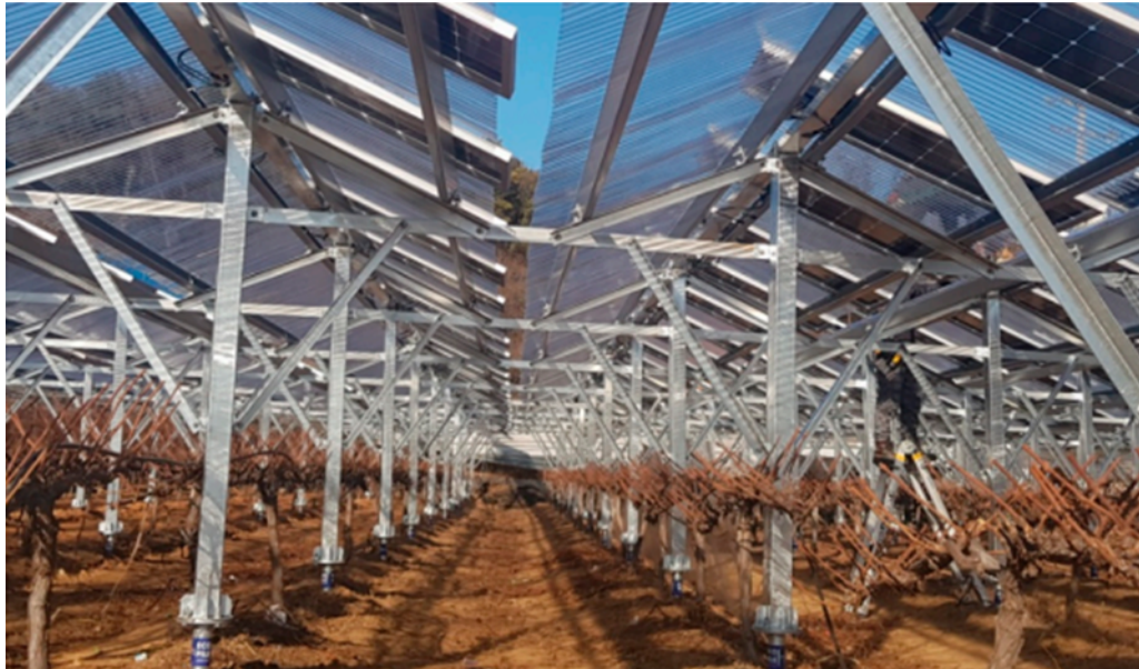
Figure 2.12: Rain-hit-protection solar facility in a grape farm.
