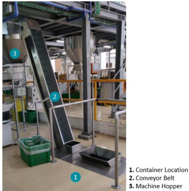
Figure 19 - Machine feeding conveyor
